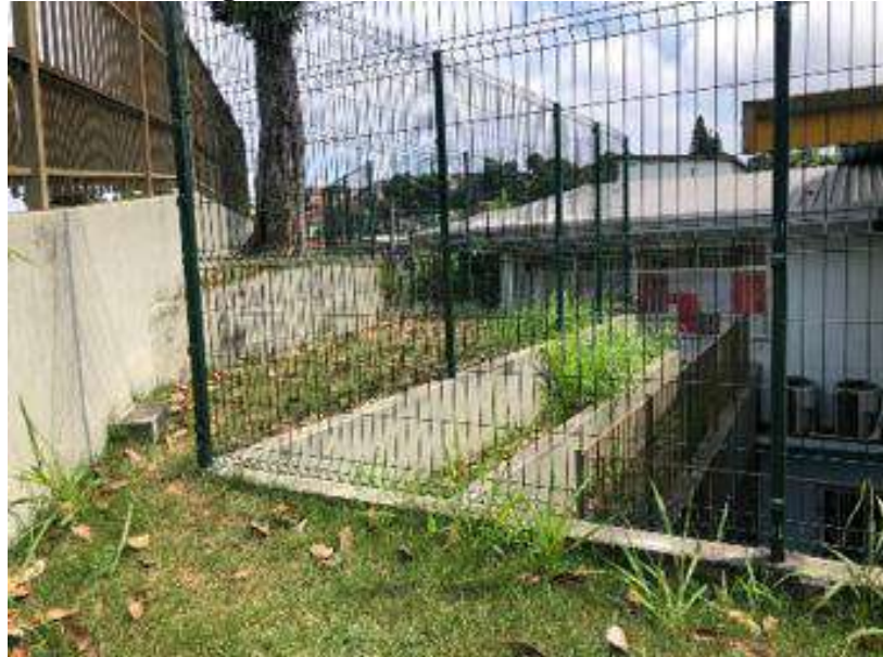
Figure 2: Installation of the Guard Rails
